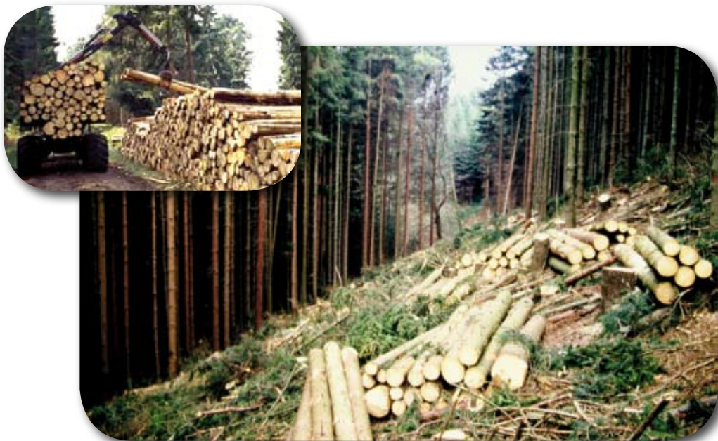
Figure 9 and 10: A major structural deficit within the forest is insufficient infrastructural development. The example from Rhineland-Palatinate shows the preparations for the construction of a new silvicultural road.
