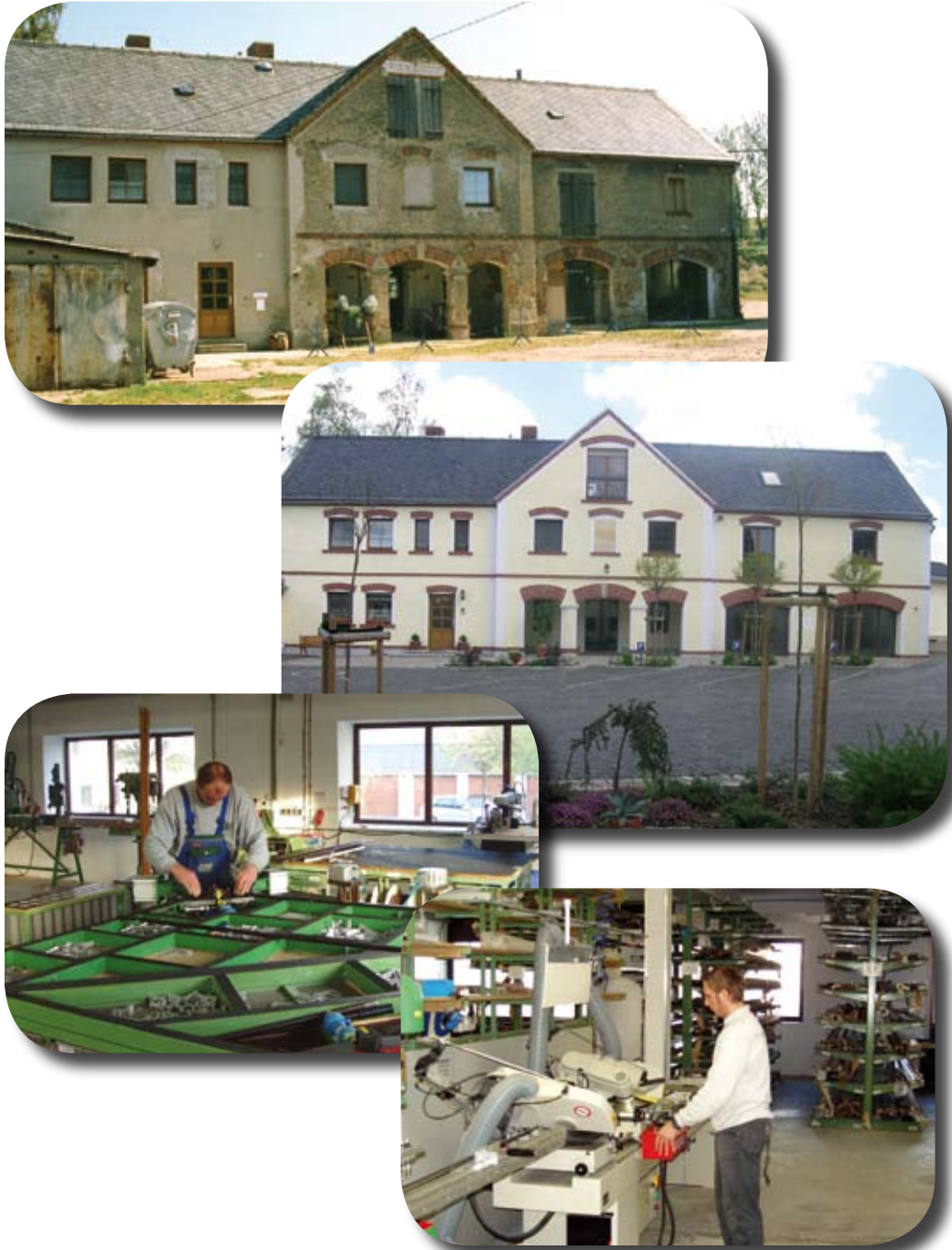
Figure 14: A historic four sided farmyard in the in the centre of Wolkau (Saxony) has been restored and converted by the enterprise Müller Systeme GmbH preserving the original character of the building. Thus, existing jobs could be maintained and new ones created.
